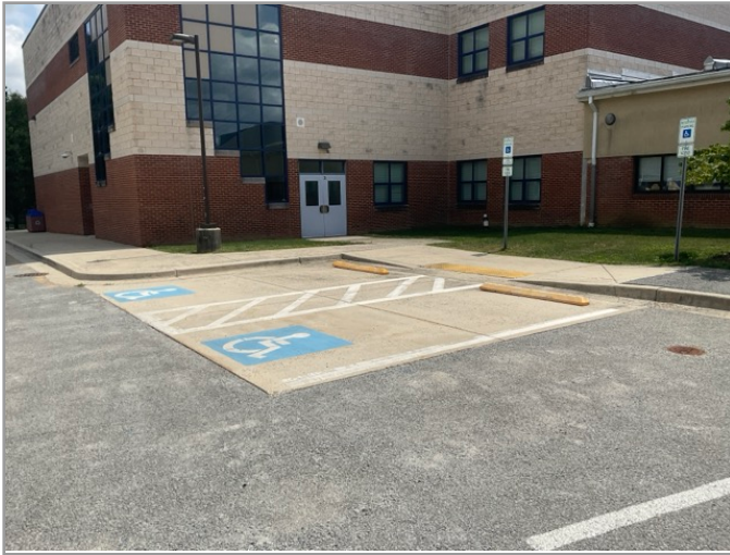
OVERVIEW OF ACCESSIBLE PARKING AREA
