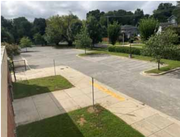
39 - SIDEWALK AND PARKING AREA
