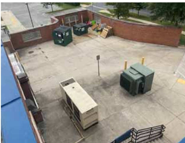
41 - SERVICE DRIVE/LOADING DOCK AREA
