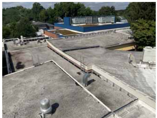
6 - OVERVIEW OF ROOF
