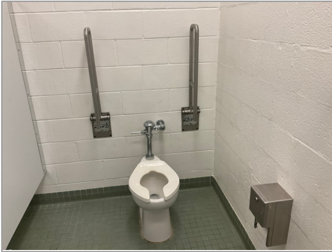
TOILET STALL OVERVIEW
